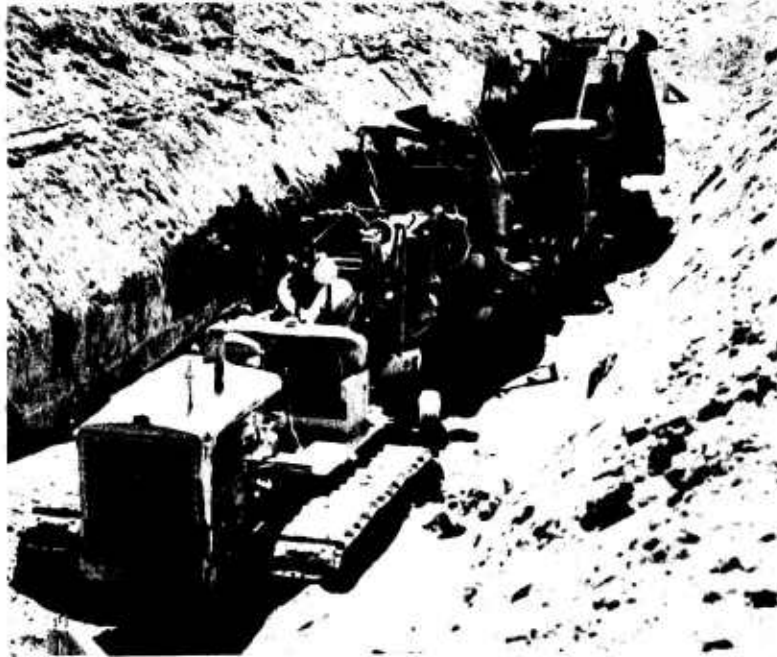
Fig. 9. Caterpillar D-7 (without attachments), 2100 ft; after test. A13327
